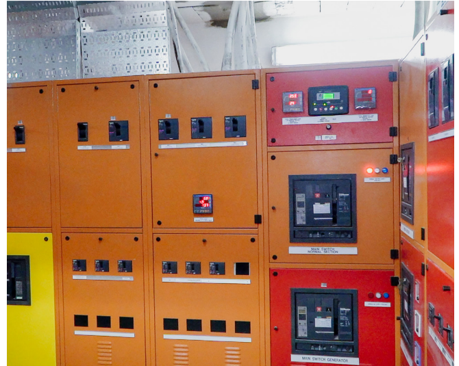
GRID-TIED SOLAR SYSTEM
